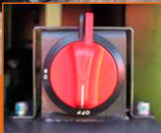
Battery cut-off switch
